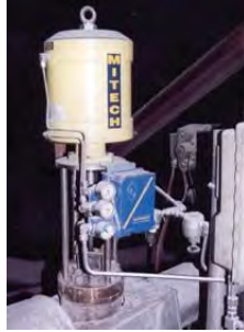
Soot Blower Valve
